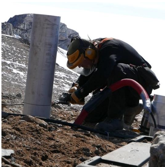
Preparation of the borehole casings for hosting the seismic sensors (left). Filling the casings with sand for insulation after installing the seismic sensors (right). Photo: NORSAR.
