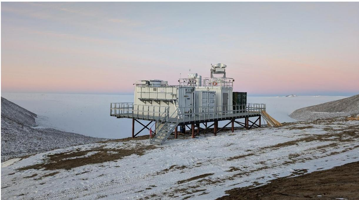
*The completed station. The weather balloon container is on the left; the hydrogen container is in the middle and the instrument/IT container is on the right; the farthest right container is used for storage. Photo: Stephen Hudson, NPI.*
